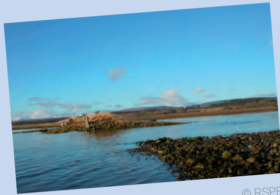
Breach in the sea wall
