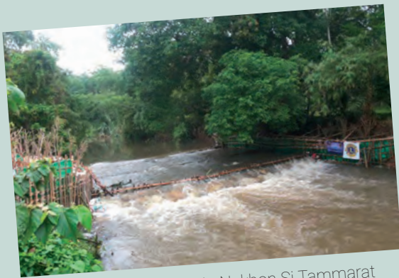
Living weir construction in Nakhon Si Thammarat with revegetation of riverbanks and bamboo structures © GIZ
