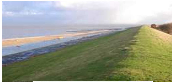
Image 2 - Coastal protection, dyke
