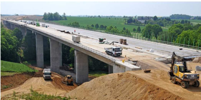
Image 1 – Bridge construction site
