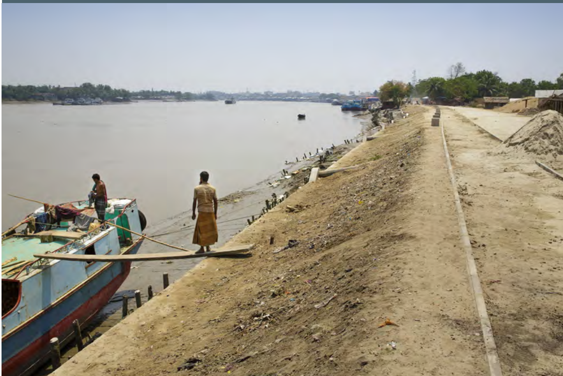
Adaptation can take various forms. Road on a dam to protect a residential district at the port of Khulna in Bangladesh.
