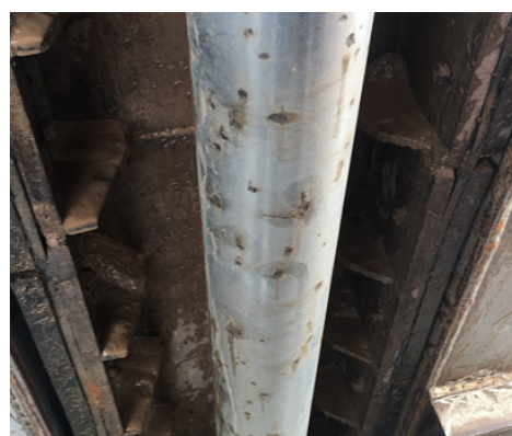
Figure 3-19. Corrosion recorded at Lang Tram gates (on the left) and hydraulic cylinders at Can Chong sluice gate (on the right)
