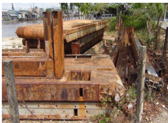
Figure 3-19. Corrosion recorded at Lang Tram gates (on the left) and hydraulic cylinders at Can Chong sluice gate (on the right)
