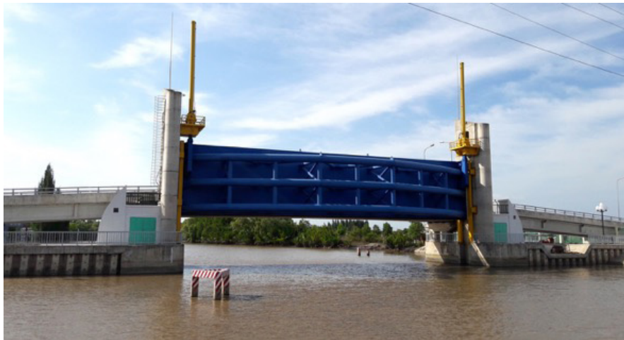
Figure 3-8. The gate of Bao Chau sluice gate (the width of 31.6 m) in Ca Mau
