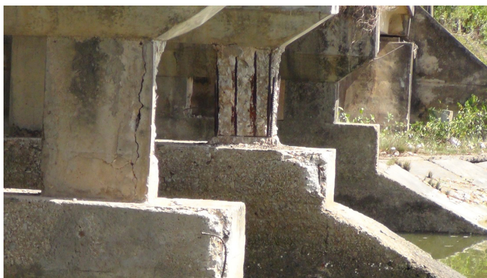
Figure 3-18. Corrosion recorded at Ho Phong sluice gate
