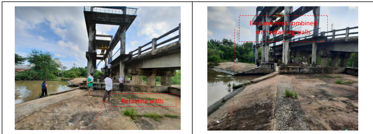
Figure 4-8. Retaining walls and connected embankment for the sluice gates in Kien Giang
