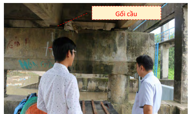
Photo of traffic bridge bearings
