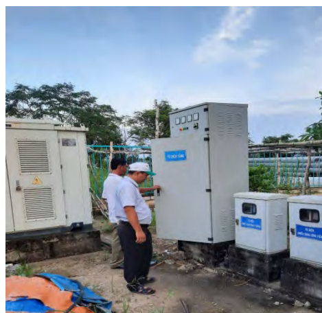
Figure 4-10. Low voltage stations, backup generators, main electrical cabinets
