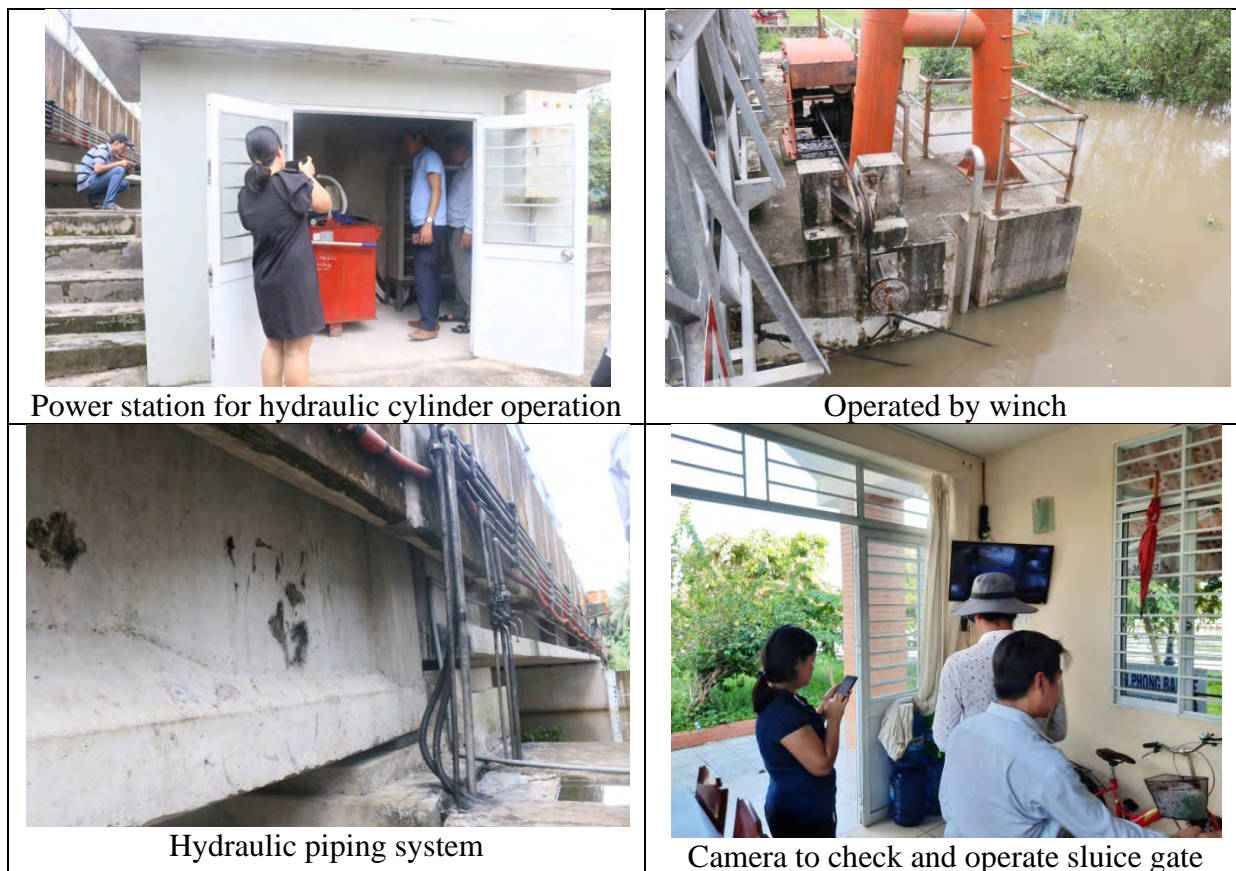
Figure 4-11. Photos of operation and control system
