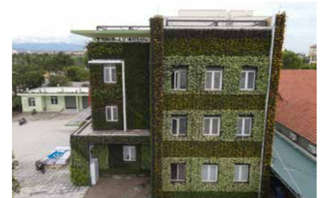
Figure 22: The left side elevation of the green wall and green roof Source: © Luong Thanh Trung/ GIZ
