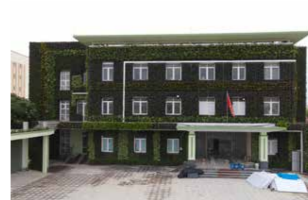
Figure 21: The front elevation of the green wall and green roof Source: © Luong Thanh Trung/ GIZ
