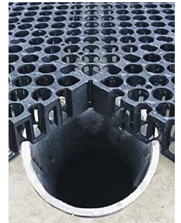
Figure 29: The plastic cup-style drainage layer of the measure's green roof Source: © GIZ/VN-SIPA Project
